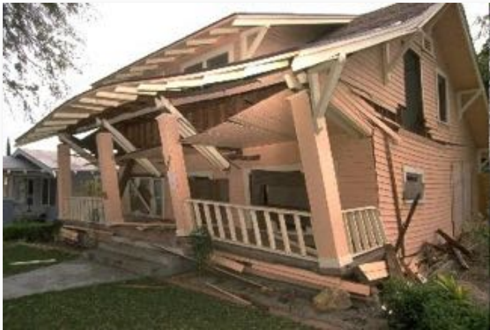
STR: Structural Drift-Sensitive
