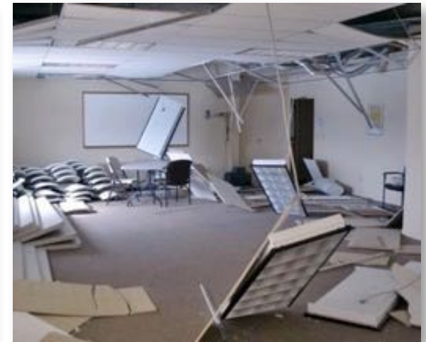
Ceilings, Equipment, Contents
